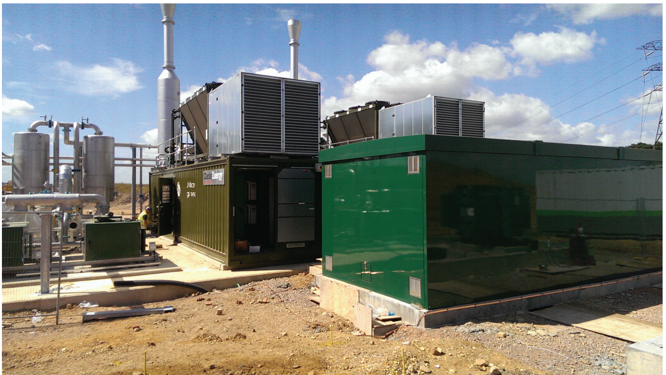
Integral to the new facility will be the engines shown above that convert gas generated by the AD process into electricity for export to the national grid
